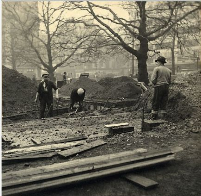
Construction of the trench shelter in Leicester Square in February, 1940 Copyright Westminster City Archives
